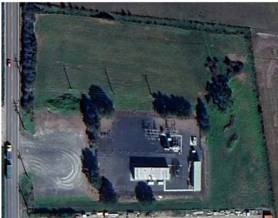
Figure 13 : Lang Lang zone substation site
