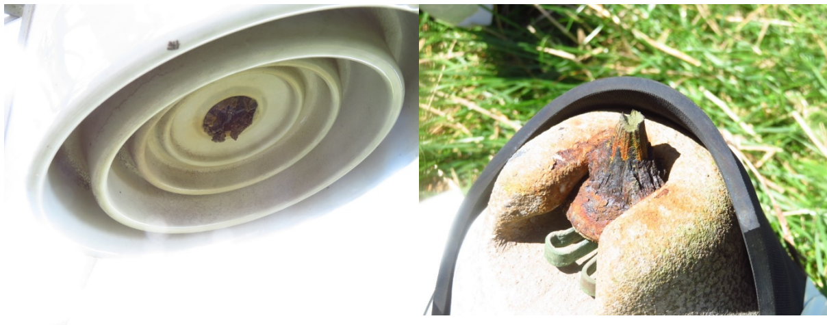
Figure 2: Severely corroded pin causing line drop
