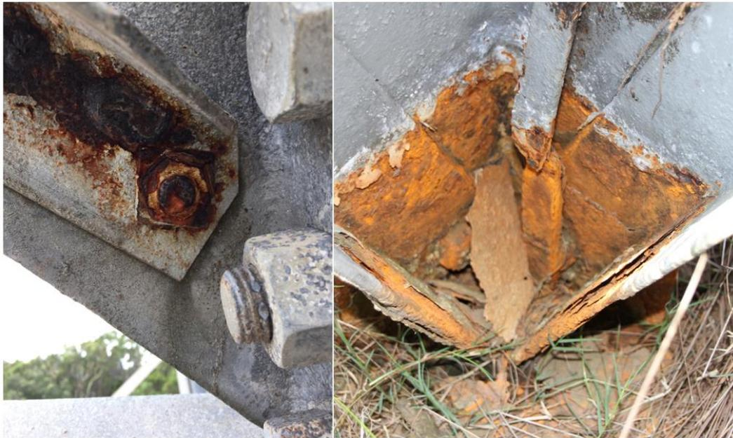
Corrosion greatly increases the likelihood of conductor drops and presents consequent bushfire risks and safety risks. While this is the case for any corroded elements of the transmission network, the bushfire risks are exacerbated for Line 25 & 26 as the lines traverse substantial sections of farmland and National Park areas. As a result, should a conductor drop occur near loose and/or dry vegetation, it can result in a bushfire, particularly if the conductor and/or line drops to the ground.
