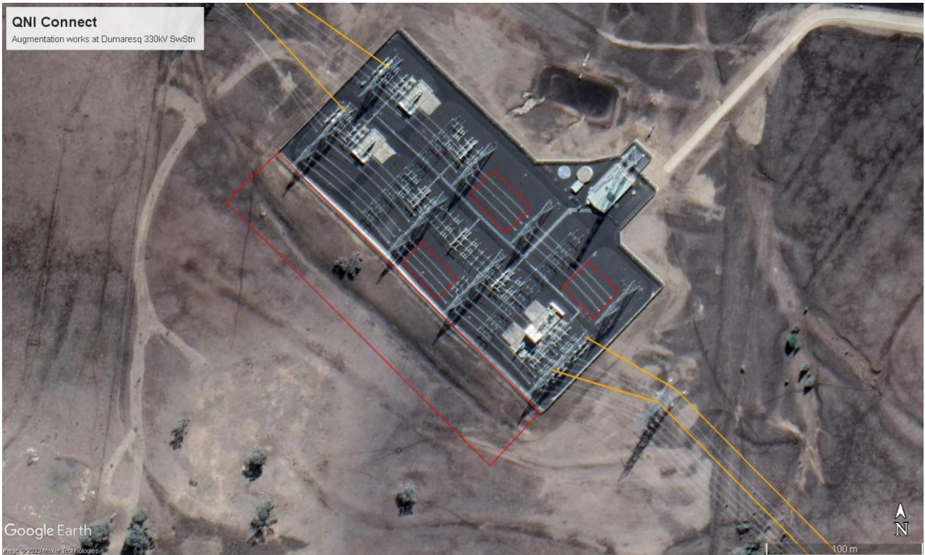
Figure 14: Dumaresq 330 kV Switching Station augmentations
