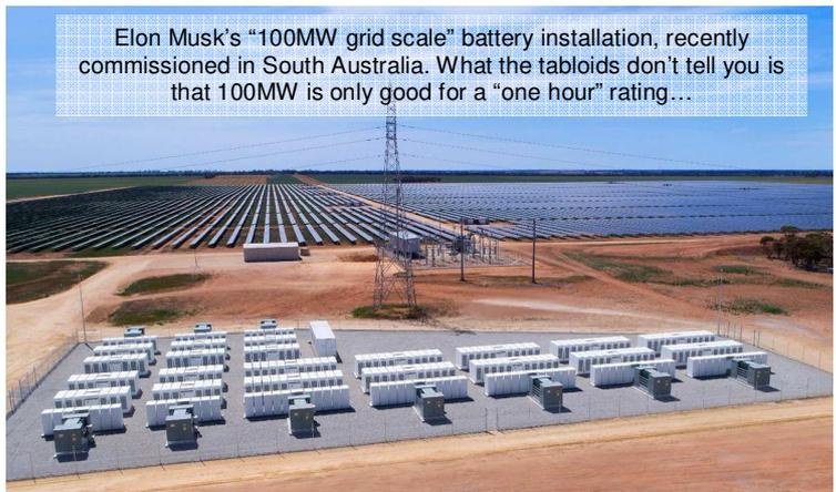
Elon Musk's “100MW grid scale” battery installation, recently commissioned in South Australia. What the tabloids don't tell you is that 100MW is only good for a “one hour” rating...
