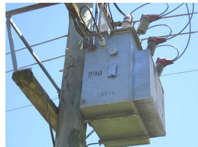
200kW distribution transformer typically feeds 15-30 houses
