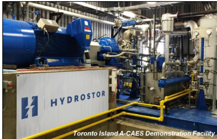
Figure 3: Toronto Island A-CAES Demonstration Facility
