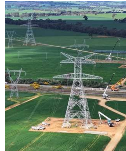
Photo: PEC under construction near Wagga
