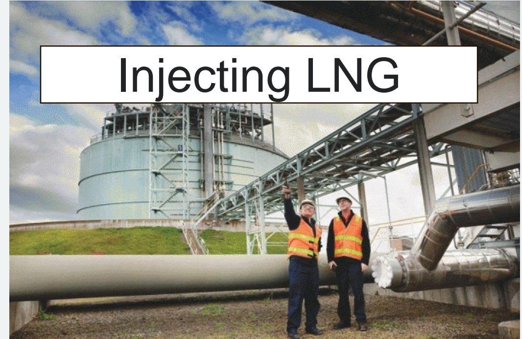
Dandenong LNG Tank, Source: The Australian Pipeliner
