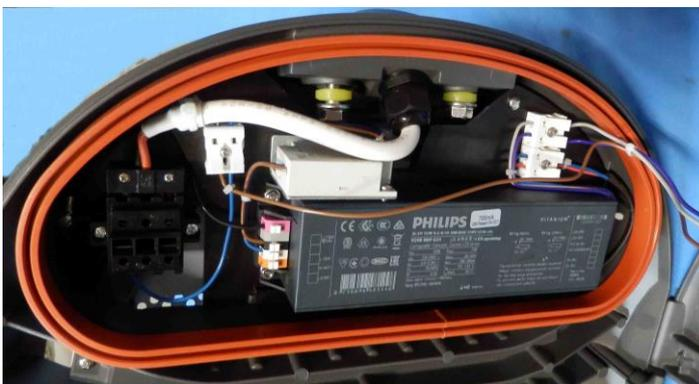
*Photo 3. Luminaire geartray.*
