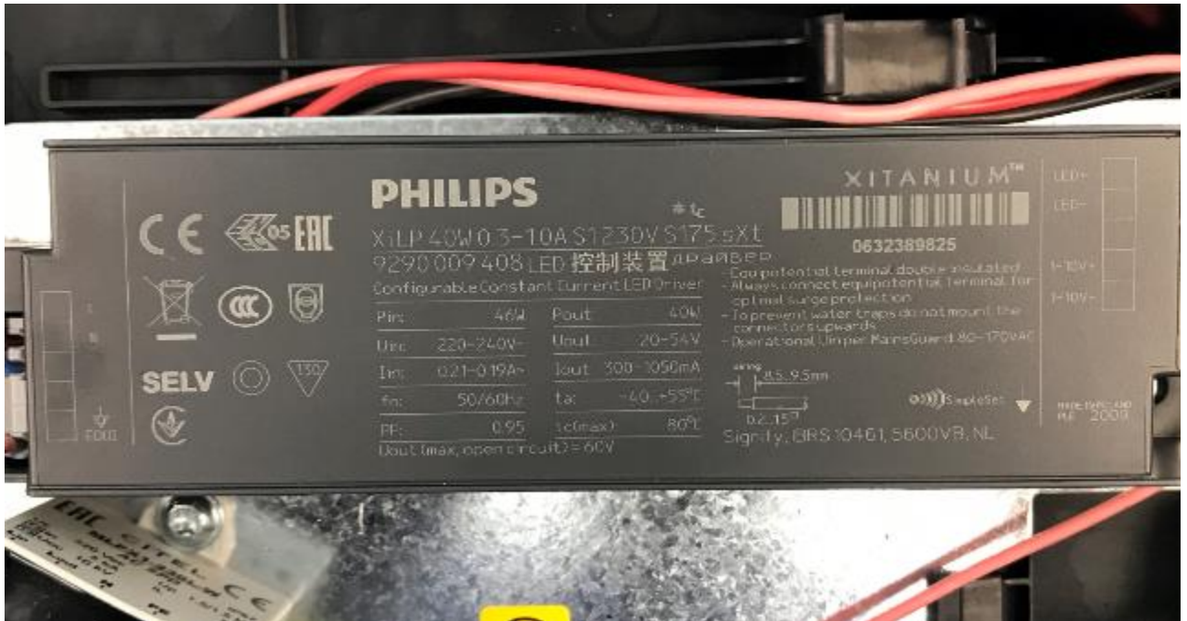
40W luminaire model - LED driver
