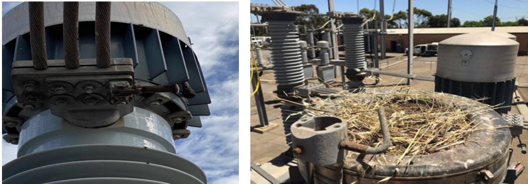
Figure 2 CT 5337 (left) and the bird's nest (right) on the top of this CT
