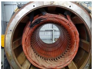
Figure 28 Damage to Mintaro diesel generator stator windings
